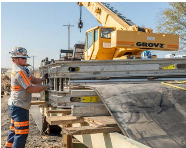
Figure 4. A belt technician tightens bolts in preparation for vulcanising.
